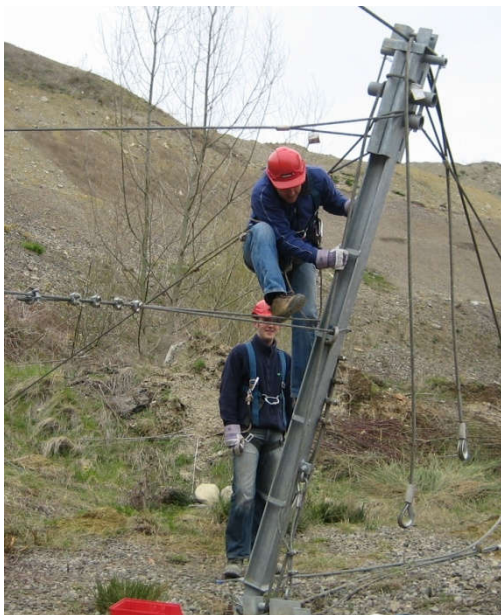
Figure 28 Tension belts between the posts for installing the nets
