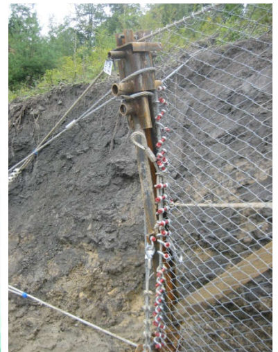
Figure 22 Vertical rope with two loops and 2 wire rope clips
