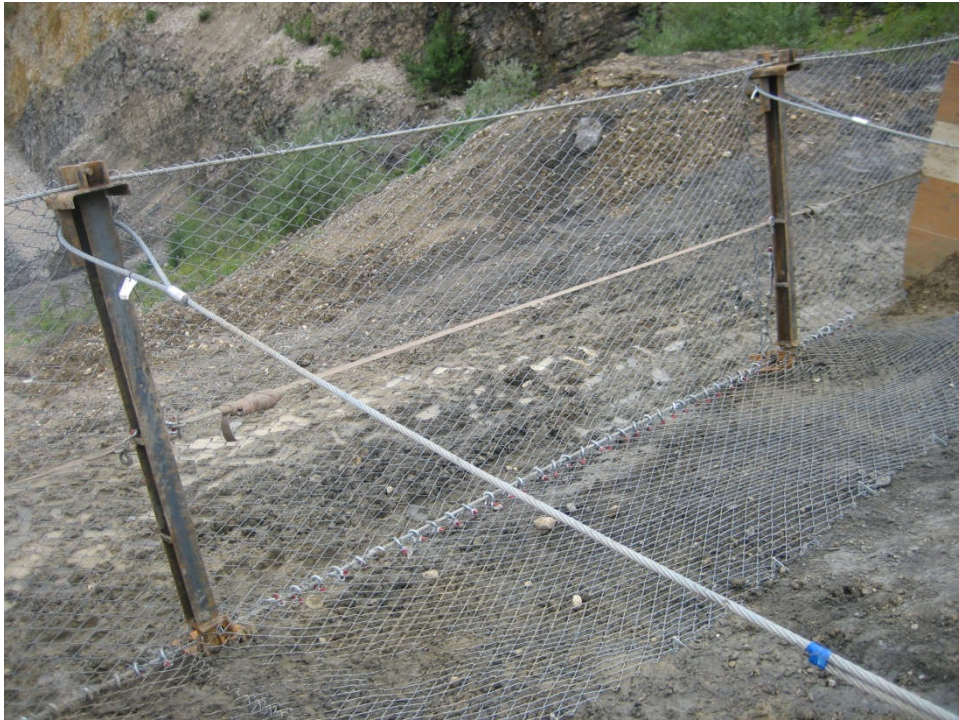
Figure 30 TECCO® mesh anchored to the ground
